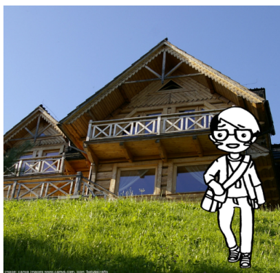
Full Exterior of the house
